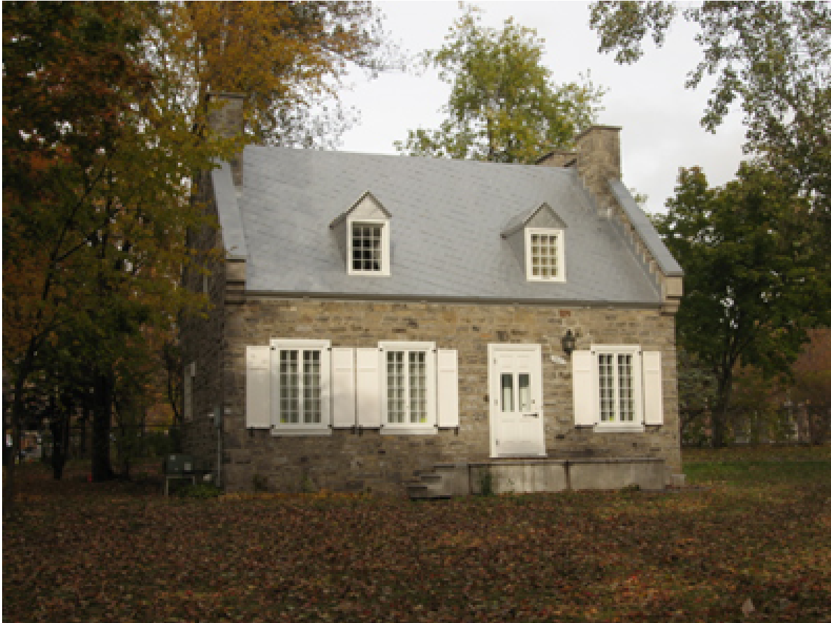
Fig. 2 Simon-Lacombe house (façade), October 2009.
