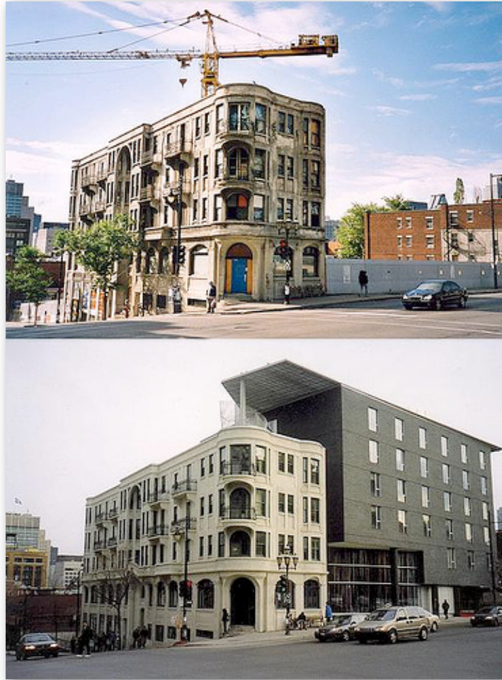
Above: The Godin Hotel (1915), Montreal, prior to 2004. Below: Hanganu Design, Opus Hotel, 2004. Photographs: courtesy of Flickr.com, 2009.
