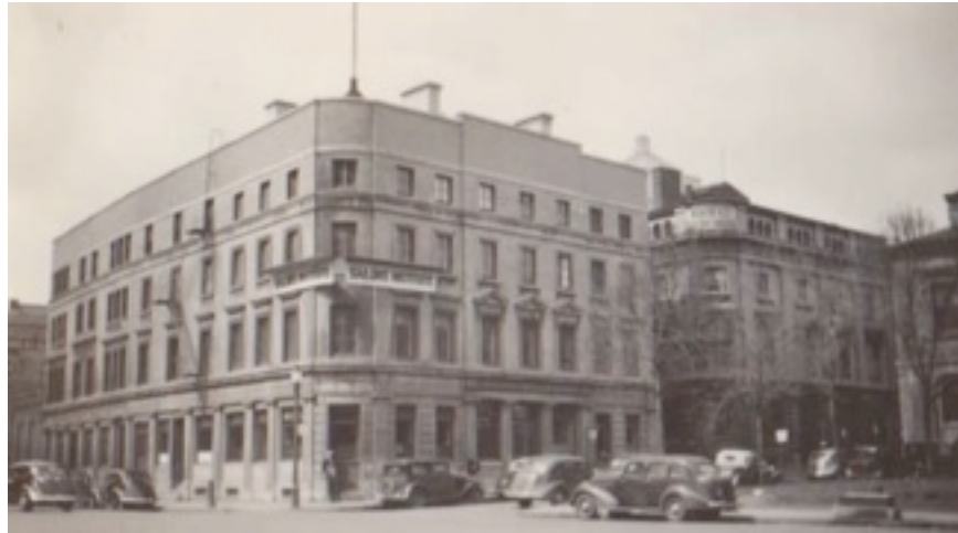
Fig. 3: The Montreal Sailors' Institute after further renovations. (Photograph of the Montreal Sailor's Institute from a scrapbook in the Mariner's House archives.)
