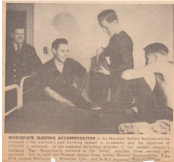
Fig. 9: A crowded bedroom at the old building for the Montreal Sailors' Institute. (Newspaper clipping found in scrapbook in the Mariner's House archives. No source information included.)
