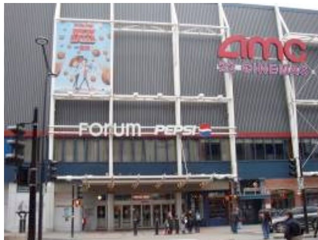
Fig. 3 Pepsi Forum façade, St-Catherine Street entrance, Montreal, 2009. Photograph: Rob Coles.
